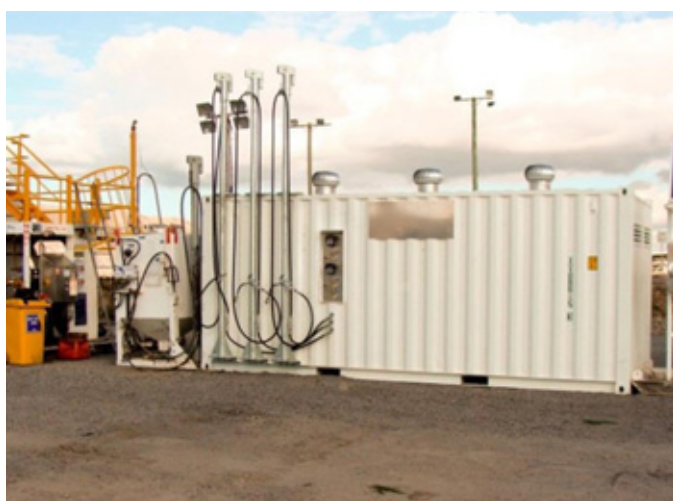
Figure 5 – Counterweighted Hose Tower
